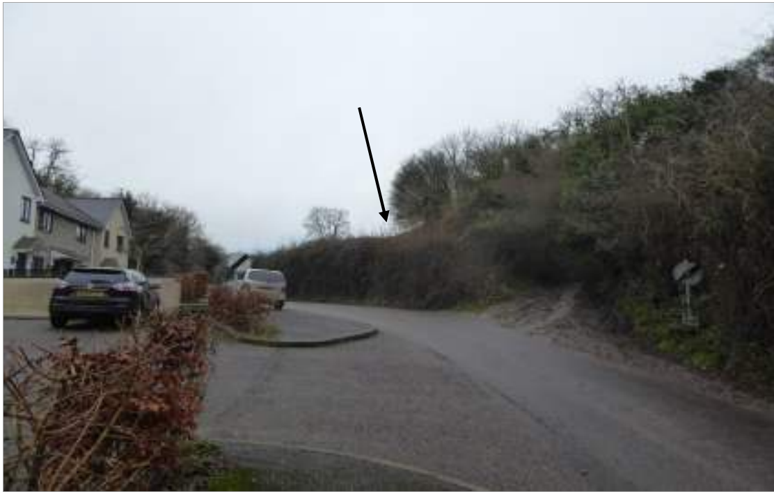
Entrance to site (below arrow) in relation to existing extremity of Beer village
